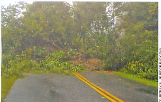
Milepost 413. This was the site of several major landslides along the parkway.
